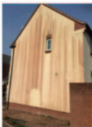
Softwashing to remove green red or black organic matter
