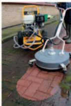
Softwashing to remove green red or black organic matter
