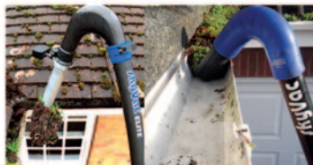
Gutter Cleaning using SkyVac high reach technology
