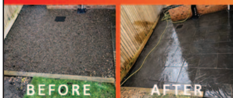
NEW PATIO INSTALLED
