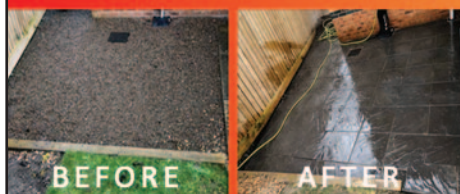
NEW PATIO INSTALLED
