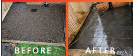
NEW PATIO INSTALLED
