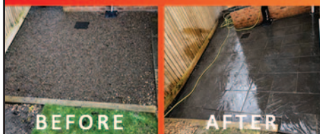
NEW PATIO INSTALLED
