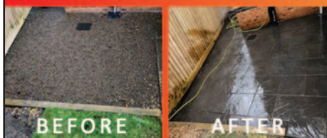
NEW PATIO INSTALLED
