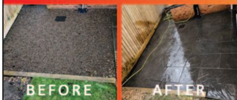
NEW PATIO INSTALLED
