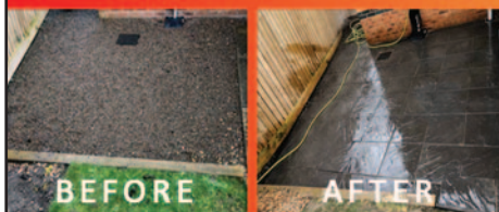
BEFORE AFTER NEW PATIO INSTALLED
