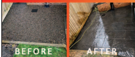
NEW PATIO INSTALLED
