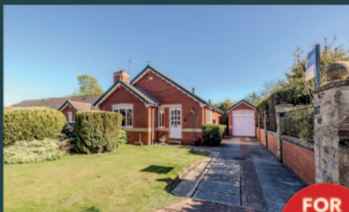
Old Station Court, Darras Hall
