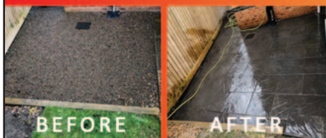
NEW PATIO INSTALLED
