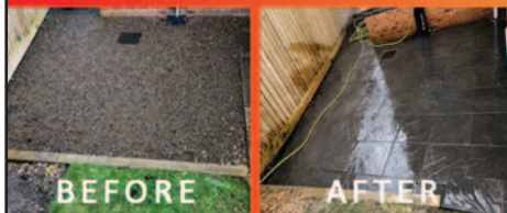
NEW PATIO INSTALLED
